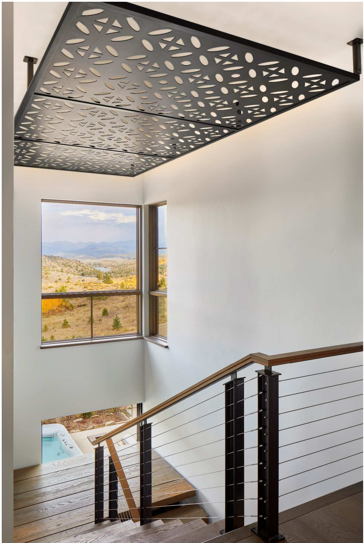
Another custom element glows upon the stair ceiling. A suspended frame cradles pierced metal panels with backlighting to create a stunning feature in what could otherwise be a simple corridor.
